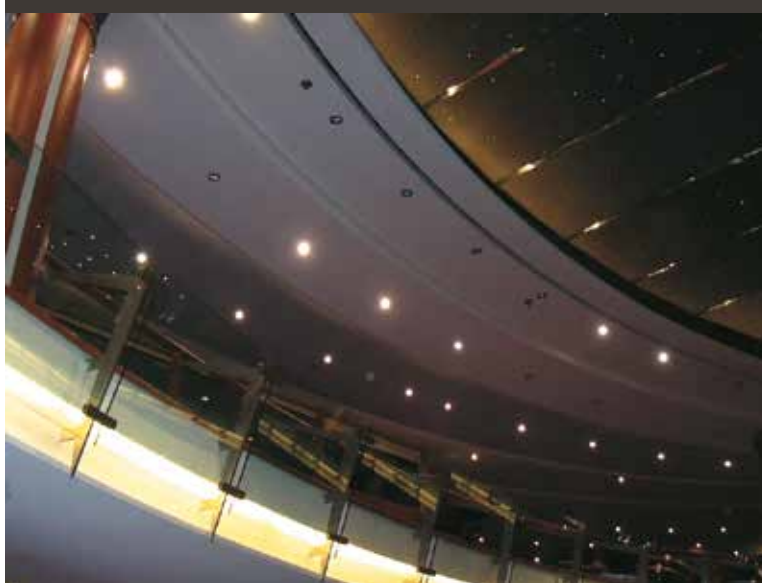
CONTROSOFFITTO HALL NAVE DA CROCIERA HALL COUNTER - CEILING ON A CRUISE SHIP
